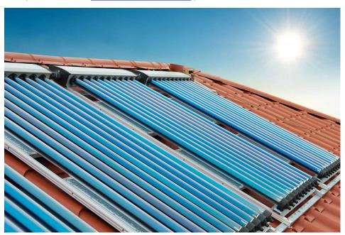
**Solar collector** is a type of solar energy panel that uses solar thermal energy. The finality of solar collectors is converting solar radiation into thermal energy. Solar energy (solar radiation) is collected by the solar collector's absorber plates. Selective coatings are often applied to the absorber plates to improve the overall collection efficiency.
